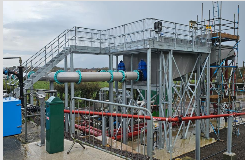
Above – Finished installation of 9m long x 3.5m wide x 5.5m high tank, pipe work with supports and access platform.
